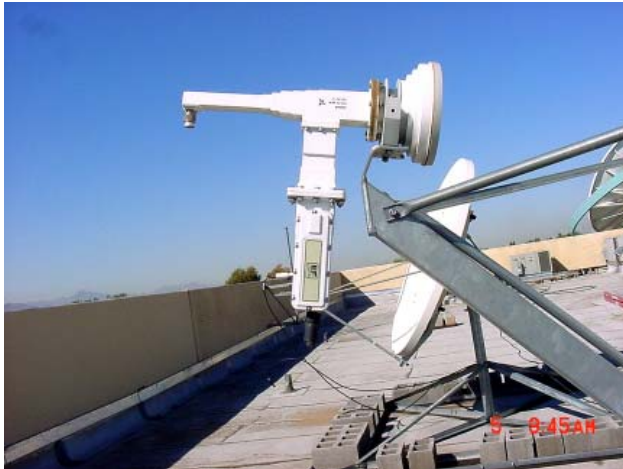
Figure B-8. Installation of LNA
