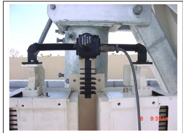
Figure B-22. Installation of the Waveguide Switch.
