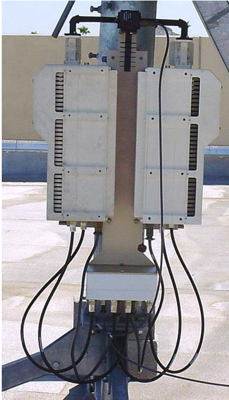
Figure B-16. Redundant Configuration
