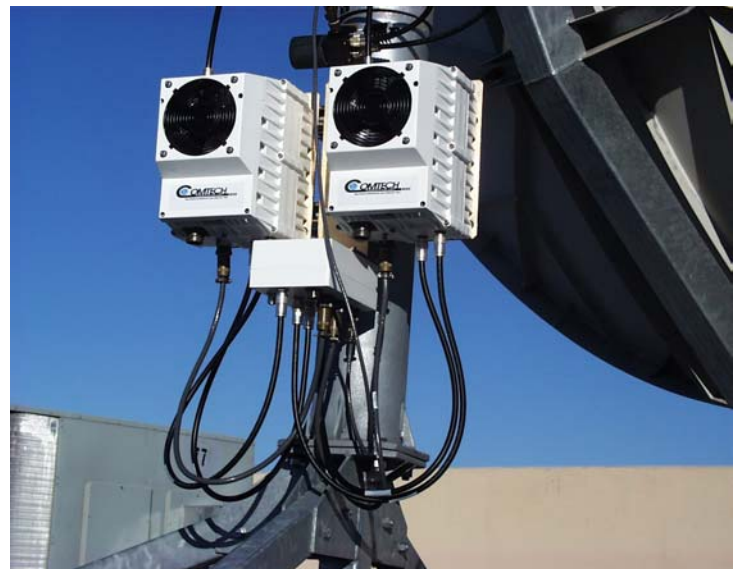
Figure A-20. Redundant Configuration with Cables Installed
