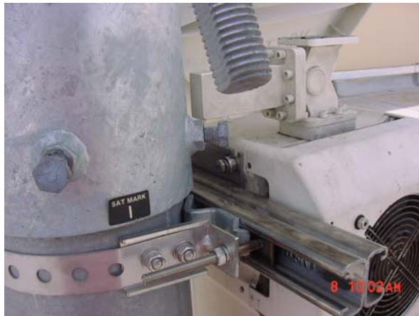
B-5. Installing the Pole Bracket
